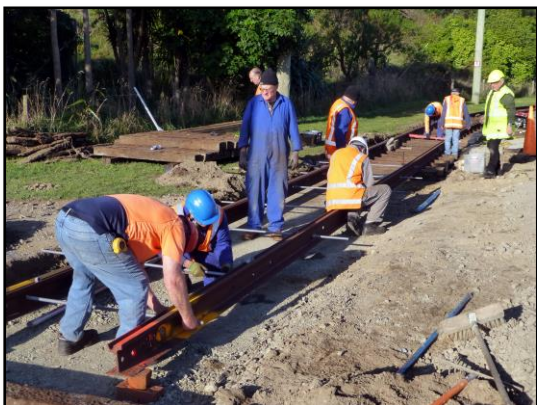
10 th June: Rails in the crossing area – installing tie-rods. Other work in background. Photo: Keith McGavin
