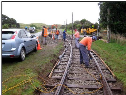
17 th June: Initial ballast spreading and packing.
