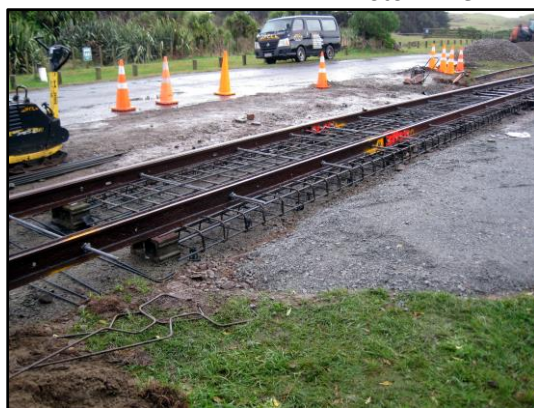
17 th June: Crossing area has been prepared for concreting by contractors. Photo: Mike Flinn
