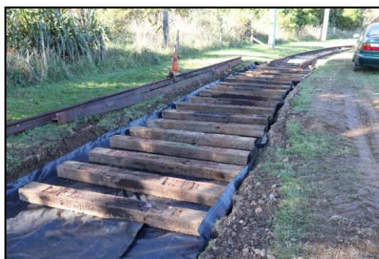
9 th June: Weed-mat and sleepers placed. Photo: Allan Neilson
