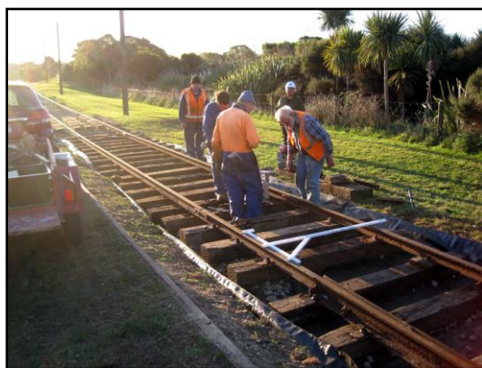
11 th June: Trackwork preparation: the transition from tramway to railway profile rail. Photo: Mike Flinn
