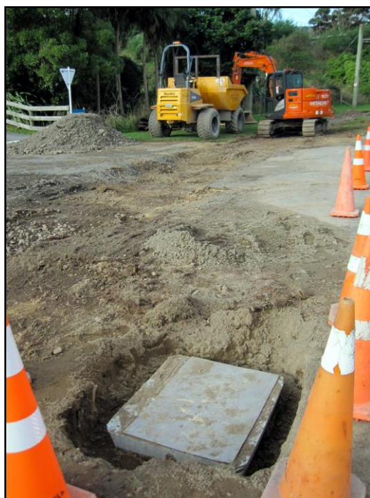
6 th June: Track-bed being prepared and drains laid by contractor. Photo: Mike Flinn
