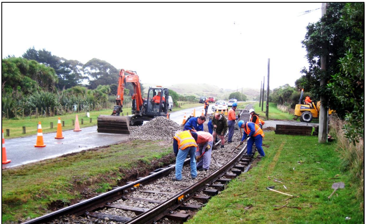
Above: Members hard at work on the road crossing track relay on an overcast and showery 17 th June. This view is looking west, towards the Beach. PCL Contractors had just arranged the ballast delivery and placement. Photo: Mike Flinn
