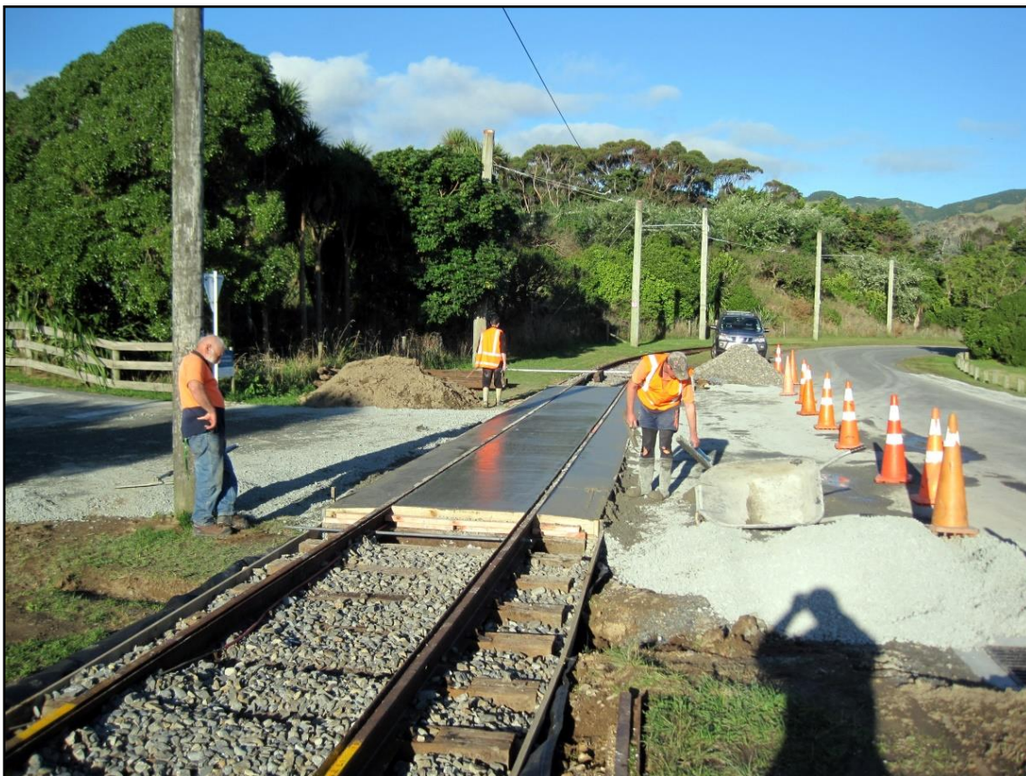
Above: Fast forward to 2020. This view shows the new crossing just after the concrete pour on 22 nd June. The four overhead poles seen on the “JAAM Tracks” cover were replaced during our 2017 overhead upgrade project and can be seen in the background. A section of the original tramway profile track is in the right foreground. Photo: Mike Flinn
