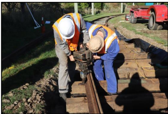
9 th June: Using the screw spike driver – rails going in. Photo: Allan Neilson
