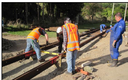
11 th June: Getting the correct crossing height and the rails level. Photo: Mike Flinn
