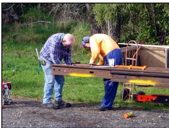
3 rd June (three photos above): Preparation of rails and fishplates, screw spikes and "A" clips etc. continues. Photos: Keith McGavin
