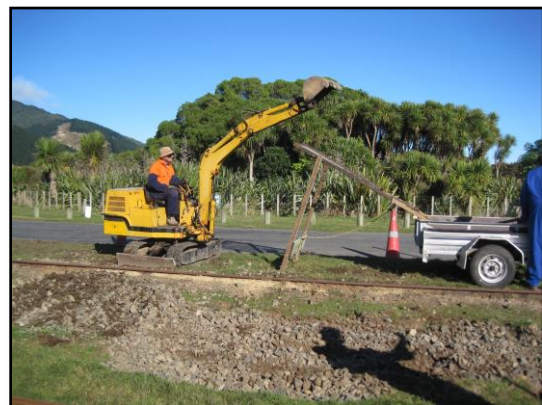
31 st May: Removal of old ballast from site Three photos above by Mike Flinn
