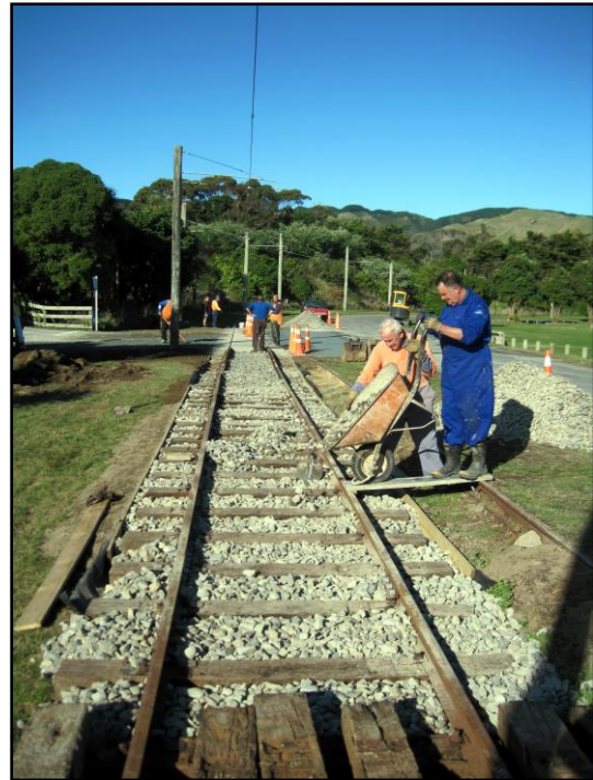
Above: Rails all connected and screw-spiked, road crossing formed and concreting complete. Track bonding, ballasting and tamping underway as the project nears completion. Looking east, back towards the tram barn, 24th June 2020.
