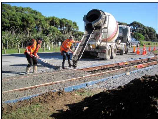
22 nd June: Contractors carry out concrete pour at crossing. Photo: Mike Flinn
