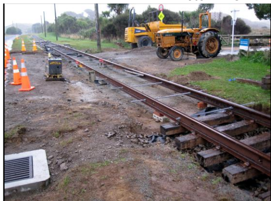
15 th June: View of the crossing area. Rails raised to correct height. Photo: Mike Flinn
