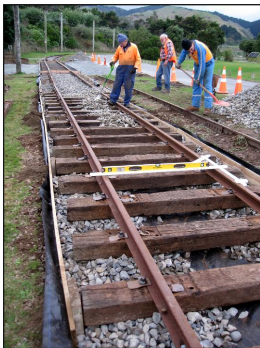
20 th June: Final rails spiked. Ballast being used to support rails to correct height.
