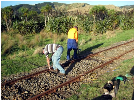
Above: Constant work continues on respiking sleepers, regauging and various other work. Here are Colin Dash (left) and Allan Neilson hard at work on 26 th April 2014.
