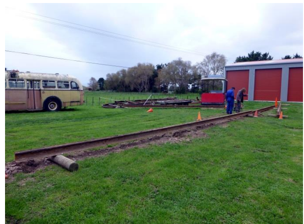
Above: A recent project has seen three disused rails, not connected to the network, lifted from the area between the barn and the rear building. Their removal will remove mowing hazards and generally make it easier to maintain a tidy back yard. The rails were part of a 4ft 8½ins gauge track used in the 1970's to move the Brisbane trams into the barn.
