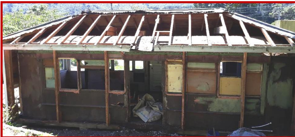
Above: Tram 86 is gradually appearing as its exterior structure is dismantled. Removal of the corrugated iron roof is revealing the original tram roof. Photo: Henry Brittain, 24 th January 2018
