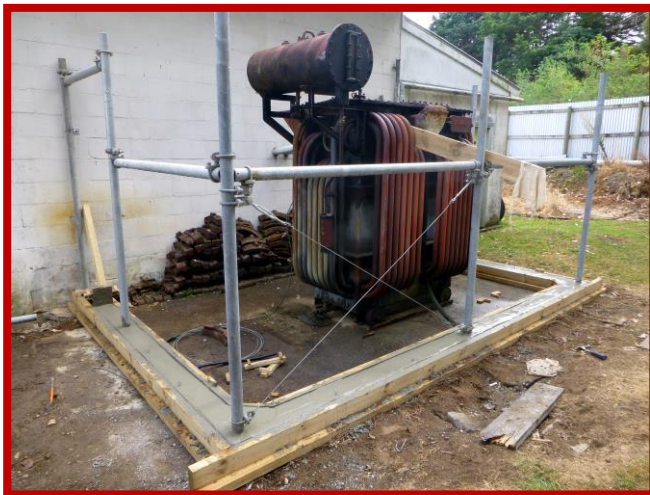
Above: New enclosure fence around the transformer being built, 17 th February 2016.
