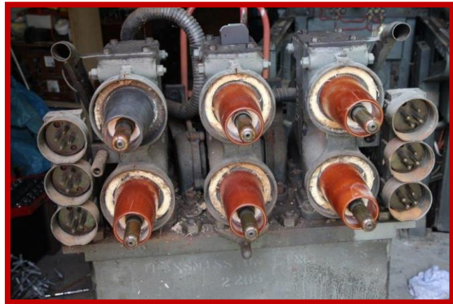
Above: OCB pin connectors – showing substantial arcing damage to the top left hand side connector.
