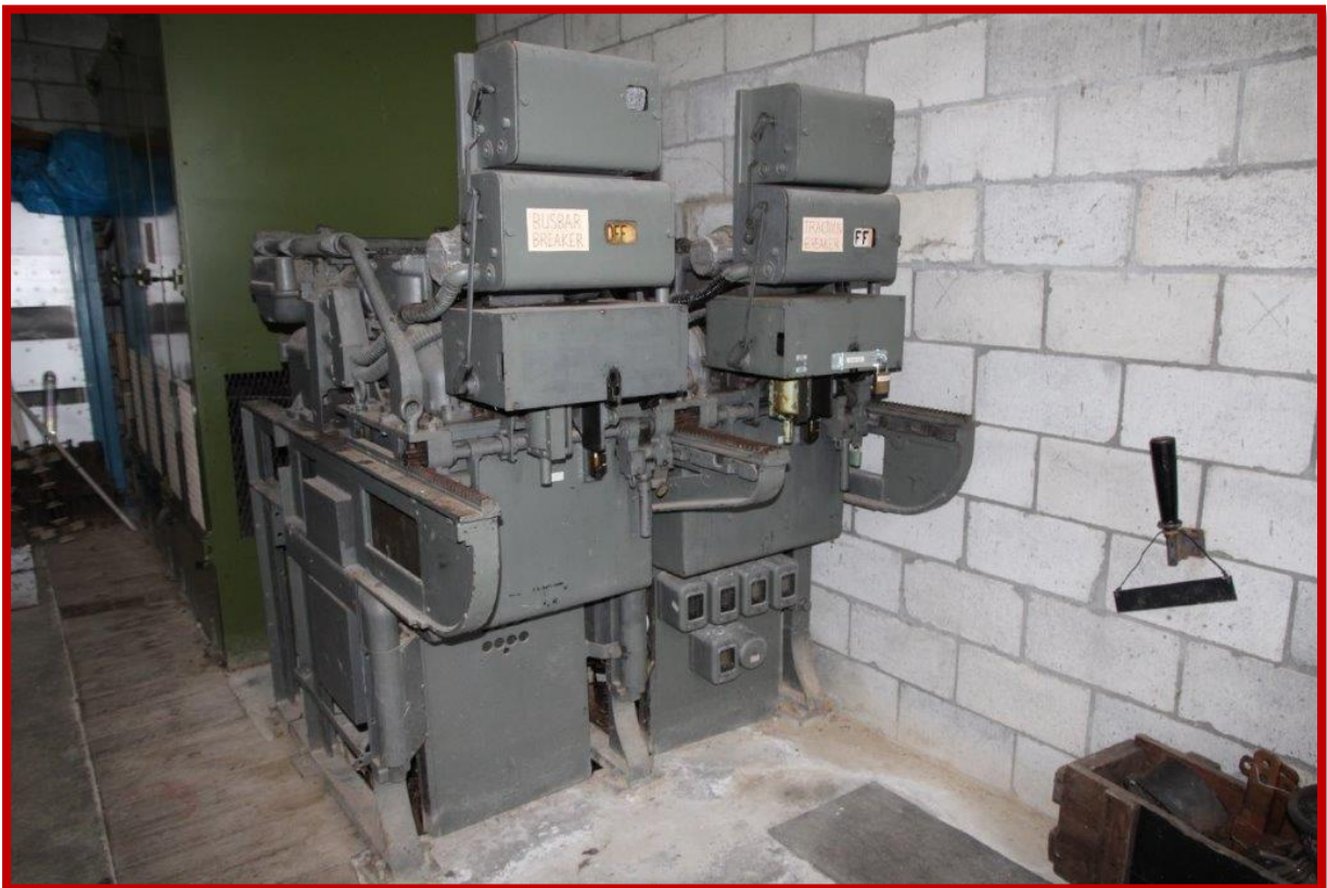
Above: The oil circuit breakers (OCB's) inside our power station. The mercury arc rectifiers are in the green cabinets in the background.
