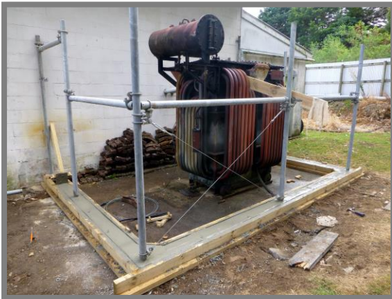
Above: A concrete nib wall was constructed around the base. 20 th February 2016.
