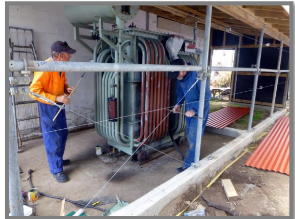
9 th March – transformer being painted. The shelter has been extended north to include a storage area.
