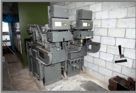
Above: The old 11kv switchgear inside the substation prior to dismantling.
