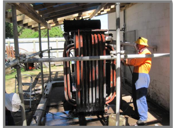
Above: By the 2 nd March the roof was in place and cleaning and undercoating of the transformer was well underway.
