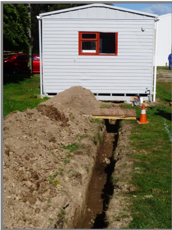
Above: Trench dug for future remote control operation of tram power from the "Palace" tea room.
