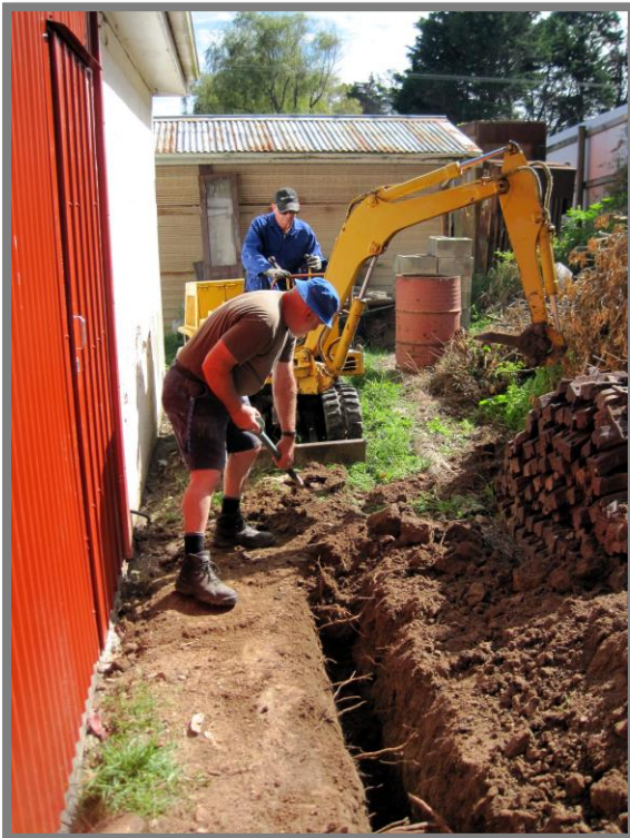
Above: Trenching for extending the earth grid, 9 th April. Steve Porter (foreground) and Colin Dash.
