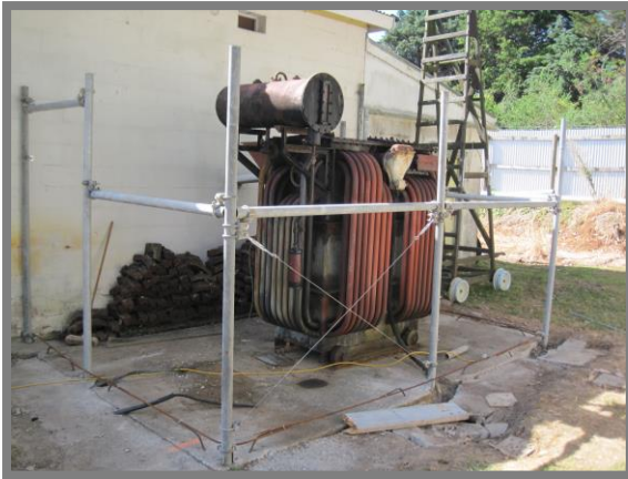
Above: By 13 th February a start had been made on the pipe fencing frame for the new transformer shelter.
