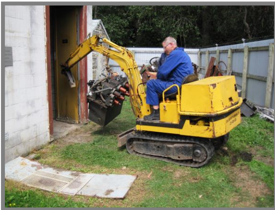
Above: Colin Dash with the Museum's loader removing part of the 11kv switchgear from inside the substation.
