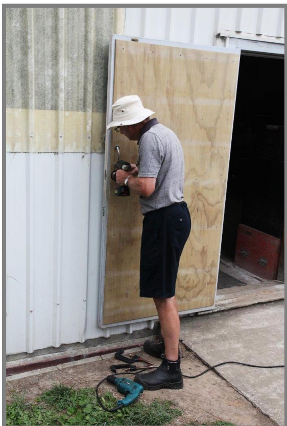
Above: Reinforcing the south workshop door and (below), assisted by Russell Jenkins, the north workshop door.
