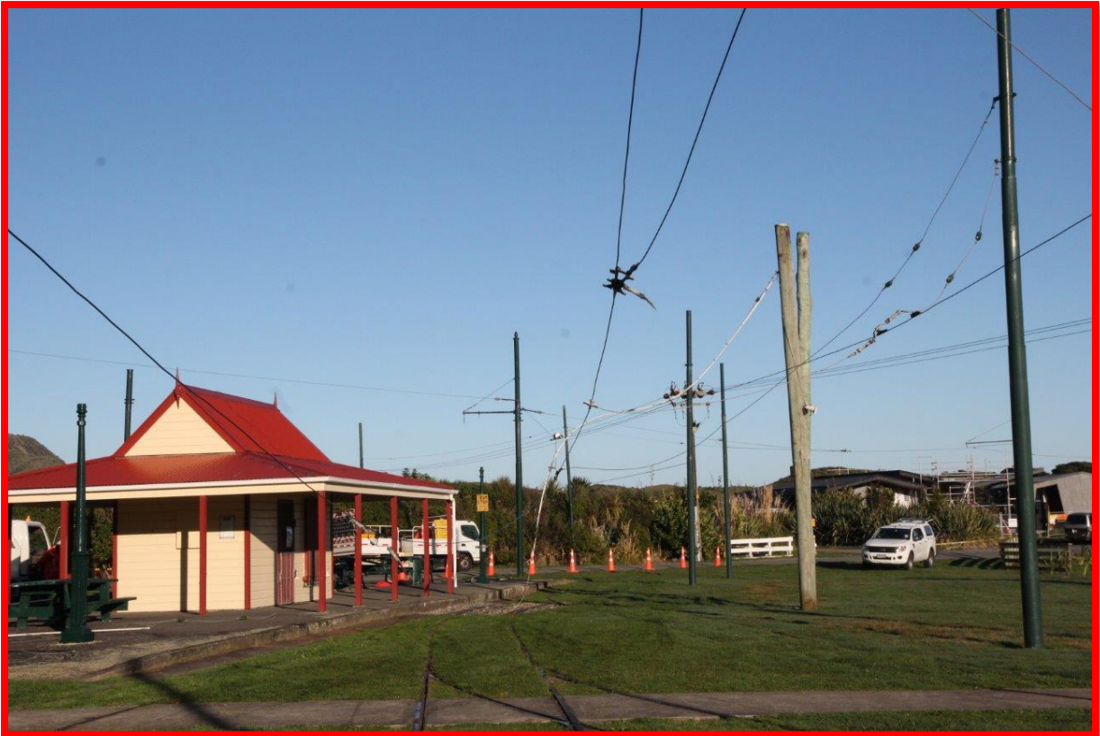
Above: The depot overhead as you have never seen it before. 16 th June 2017. In case you are wondering the whole of the depot overhead running wire and span wire is being replaced.
