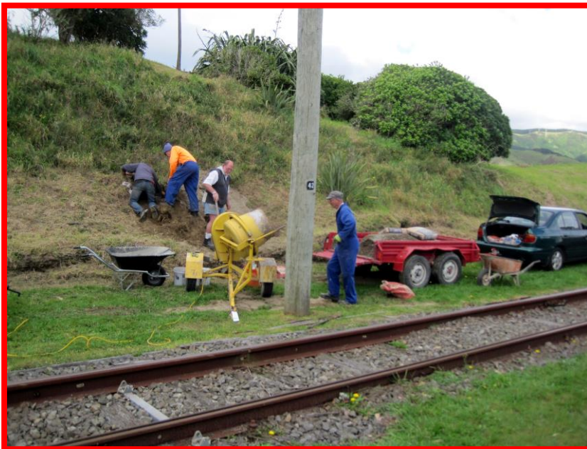
Above: An anchor for pole 42 had to be concreted in part-way up a bank, 19 th April. Members in this photo are, from left, Murray Gibson, Allan Neilson, Phillip Austin and Colin Dash. Photo: Mike Flinn
