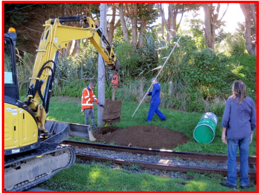
Above: Auguring one of 17 holes 18 th April. Colin Dash in background with the "hole depth measuring device". Photo: Mike Flinn
