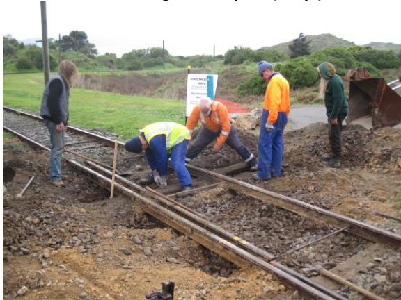
2. Below: Removing old sleepers (Easy!)
