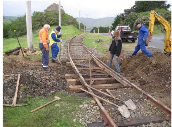
3. Above: Sliding new sleepers into position (Easy!)
