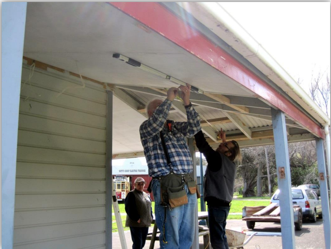
Above: Steve Porter and Murray Gibson busy fixing plywood panels to form a veranda ceiling for the platform shelter / kiosk. Marlene Wilson looks on.
