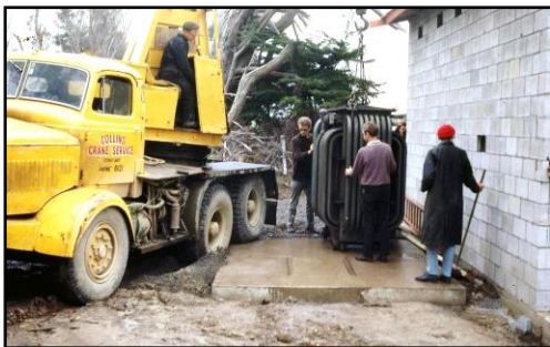
Above: Installing the 11kV transformer.
