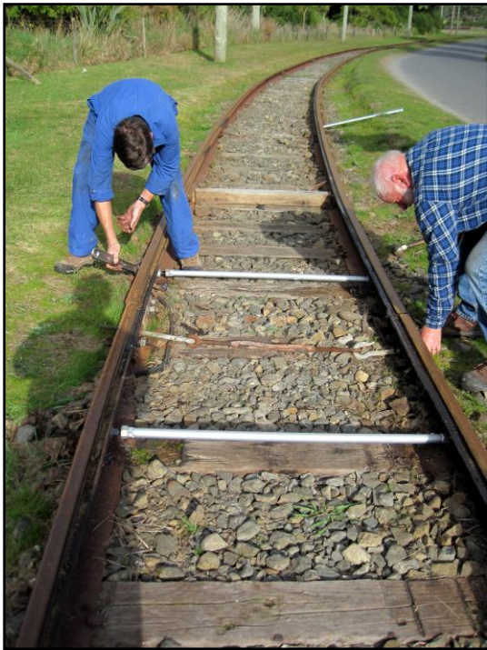
Above: New pipe-type tie-bars being installed, 5 th August 2020.
