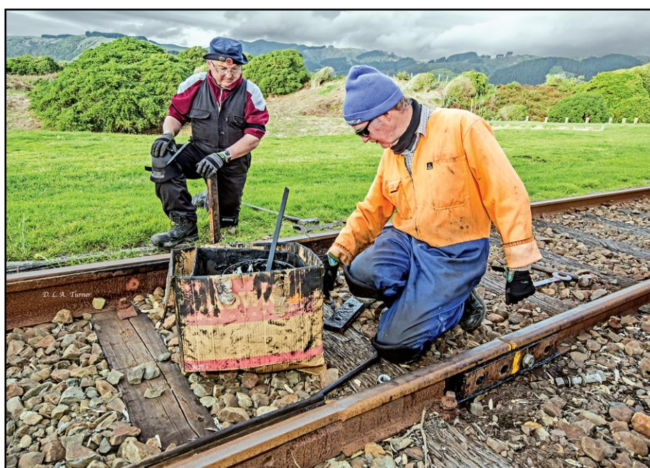
Left – A photo by Dave Turner of trackwork (rail joint maintenance) on the Kāpiti Coast Electric Tramway.
