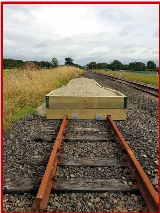
The sand trap built by WRPS to KiwiRail requirements and the cut made in the track that used to connect the KR loop to the WRPS line. The line on the right is the Marton – New Plymouth main-line at Lepperton.
